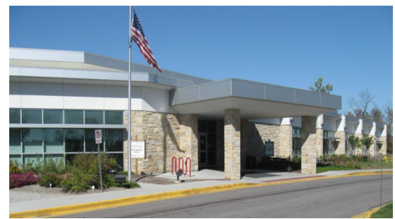
Southeast Community Center in Kansas City, Missouri
